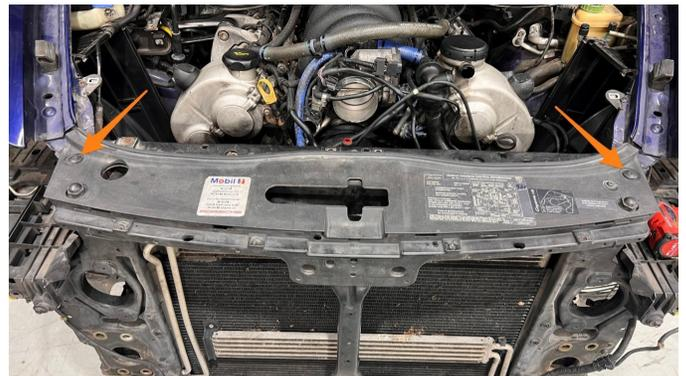
**46.** Remove upper rubber seal and mounts.
